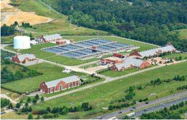
Griffith Water Treatment Plant
