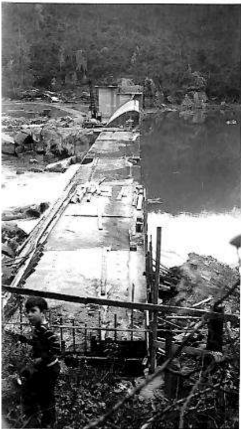
Construction of the Low Dam, 1950
