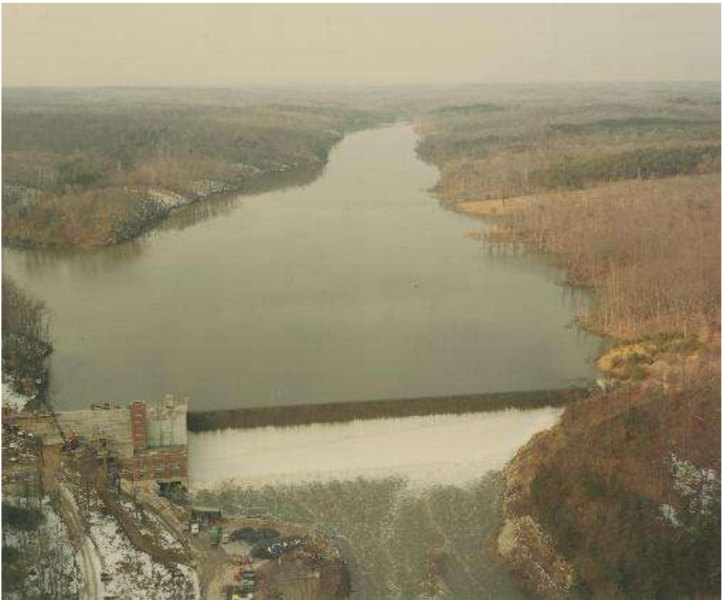
Full Reservoir at High Dam, 1960
