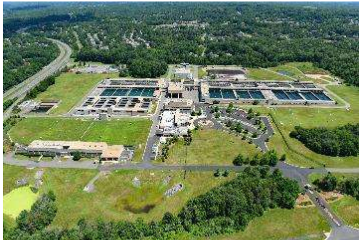
Corbalis Water Treatment Plant
