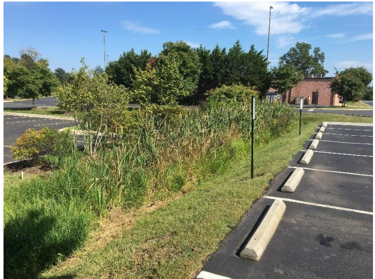
Figure 5-19. Bioswale to catch runoff from parking lot, Marshall, Virginia (September 2016).
