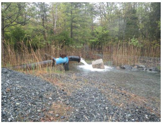
Quarry sump discharge at the surface above west quarry rim.
