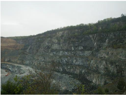
Benched SW highwall. Slide plane evident in bench. Mining actively occurring at base of wall.
