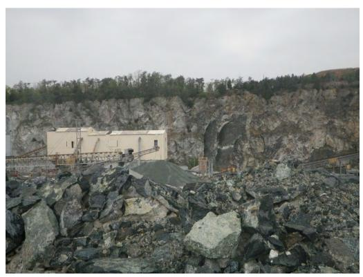
NW highwall with rock wedge (dogtooth) failures along joints in back wall.
