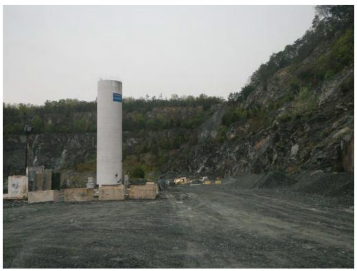
Water tank holding quarry sump water for dust control use.
