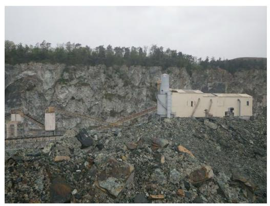
NW highwall with rock wedge failures visible.
