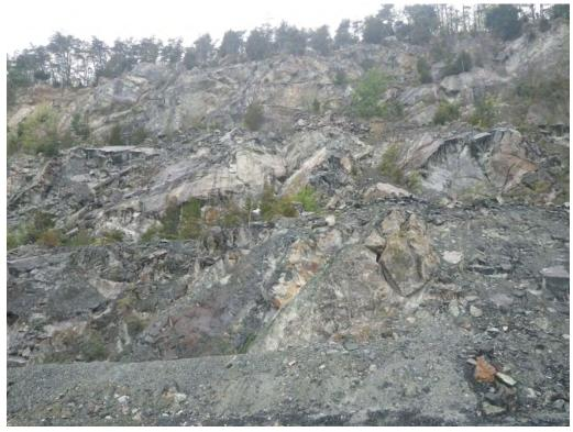
Blast damaged southern end of NW highwall.
