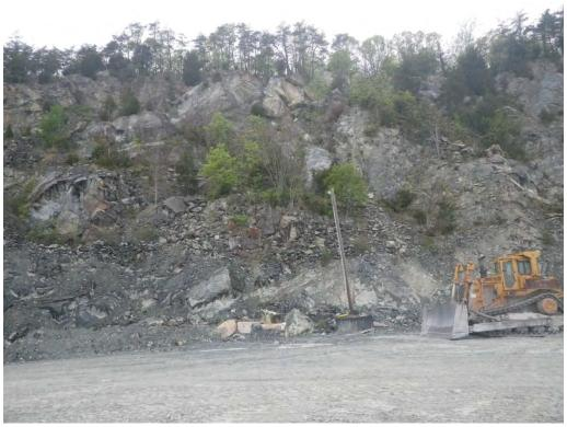
Southern end of NW highwall. Undefined rock benches with blast damage induced rock falls.
