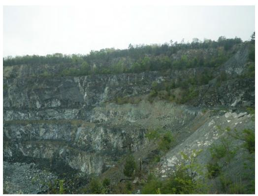
West end of SW highwall. Slip plane is visible.
