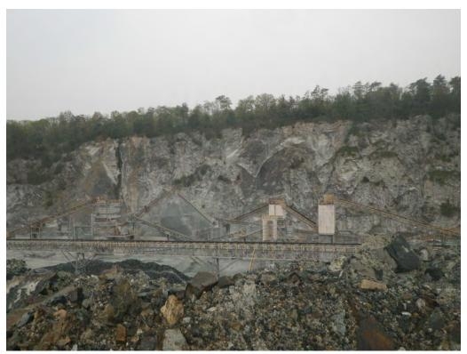
NW highwall, minimal soil cover present above rock. Black staining from surface water flow.
