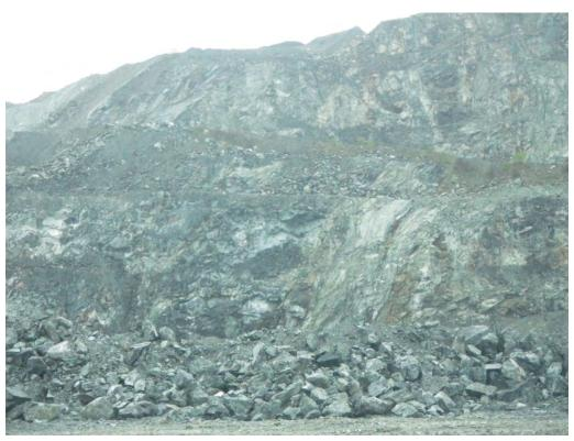
NE highwall. Blast damage evident.
