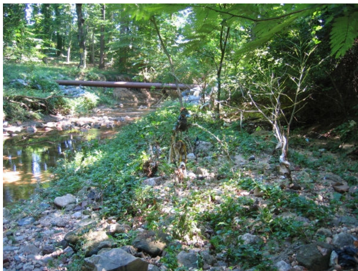
14-002A: View looking down stream at trash on trees and exposed pipe crossing stream
