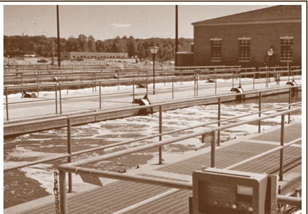
Settling basins at Blue Plains Regional Wastewater Treatment Plant. Nitrogen reductions scheduled for the plant will reduce the loading from the largest point source of nitrogen on the Potomac.
