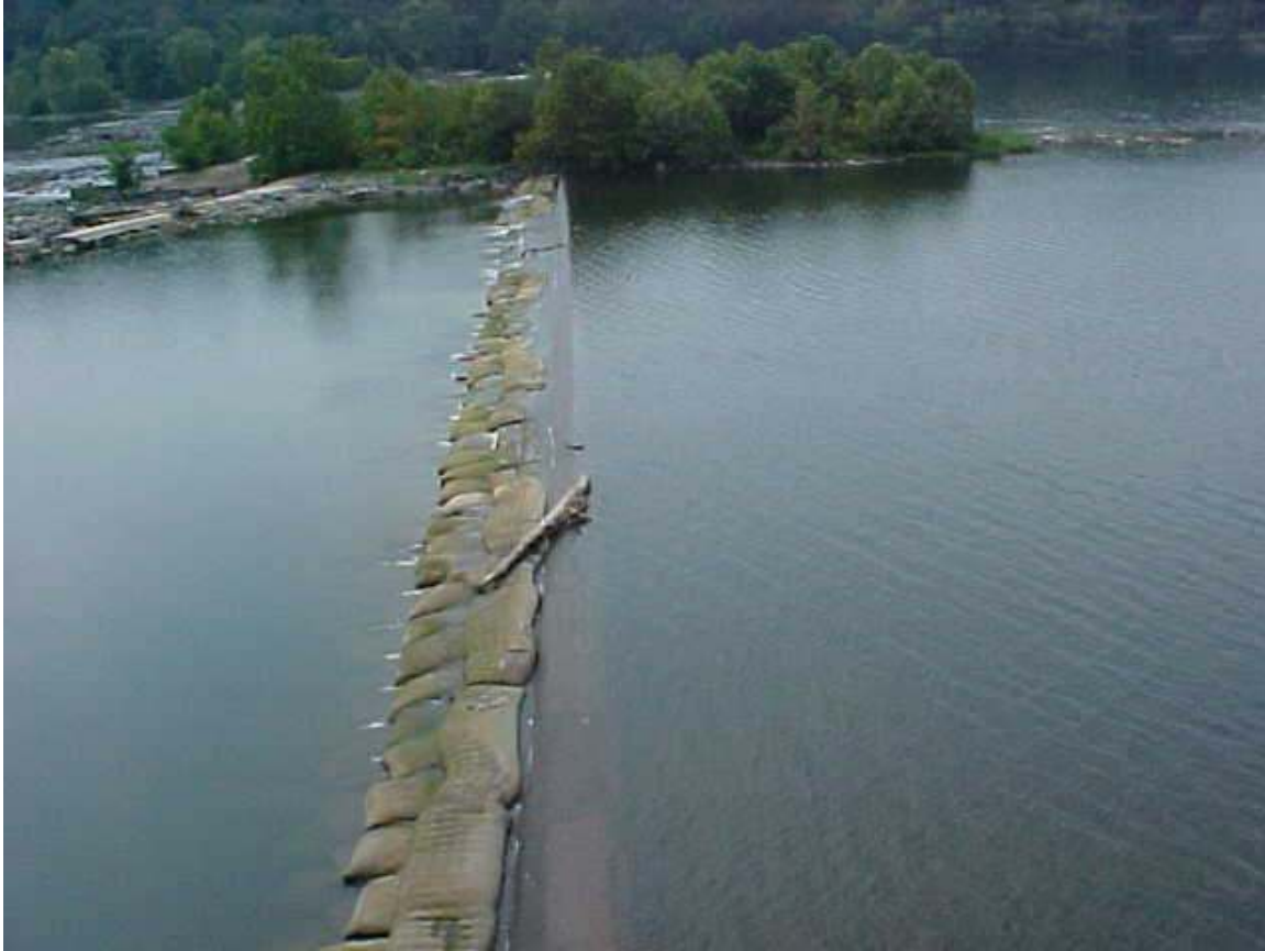
Photo credit: Woody Peterson, Washington Aqueduct. View towards Snake Island from the balcony of the Little Falls Intake during low flow conditions on August 19, 2002 (flow of approximately 170 mgd)
