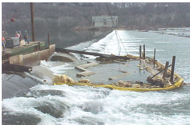
Figure 1: The Little Falls Fishway, nearing completion in January 2000, the 28' notch and "W" shaped weirs are visible. The USCOE pumping station and Maryland shoreline are in the background. Photo by Nancy Jedziniak, USCOE.
