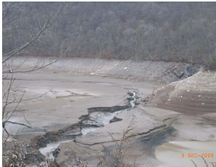
Figure 1 Photo of the drained Savage River Reservoir showing the beginning of a channel being cut by run-of-the-river flow.
